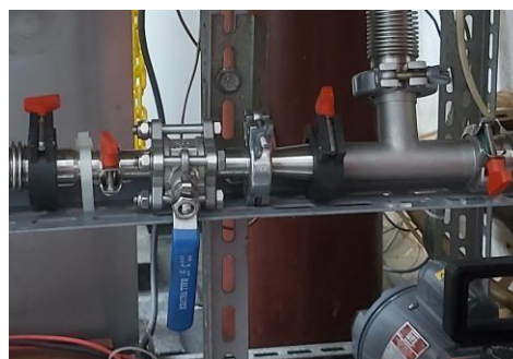
Fig. 6. The ball valves were replaced with new stainless steel ones. All connections and clamps are new.
