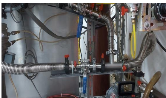
Fig. 5. All bellows were replaced with new ones. The system no longer has rubber hoses and copper pipes.
